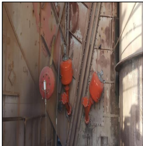
Installation of Air Blasters
